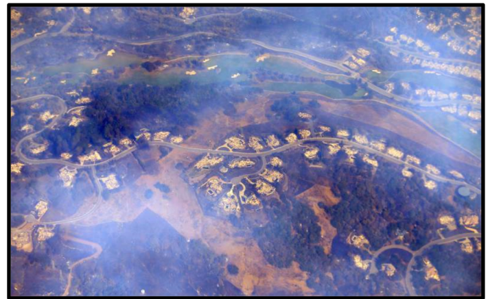
Santa Rosa 2017 aerial photo shows open space unburned with homes burned to the ground.
